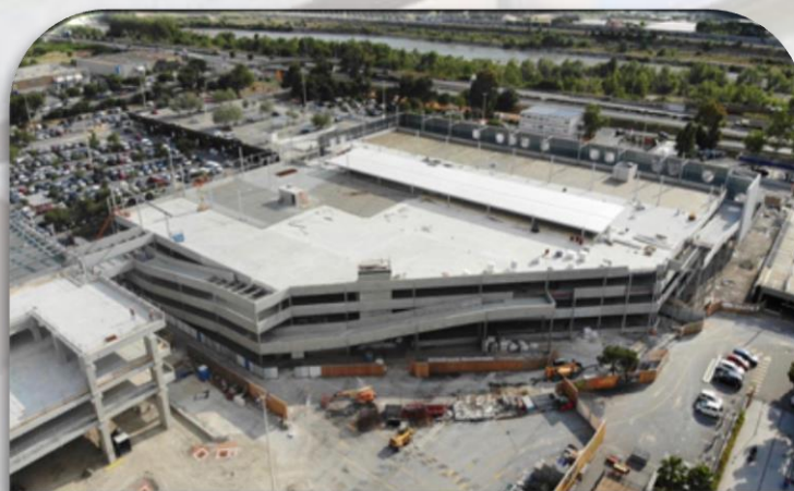
Chantier Parking Carrefour Nice
